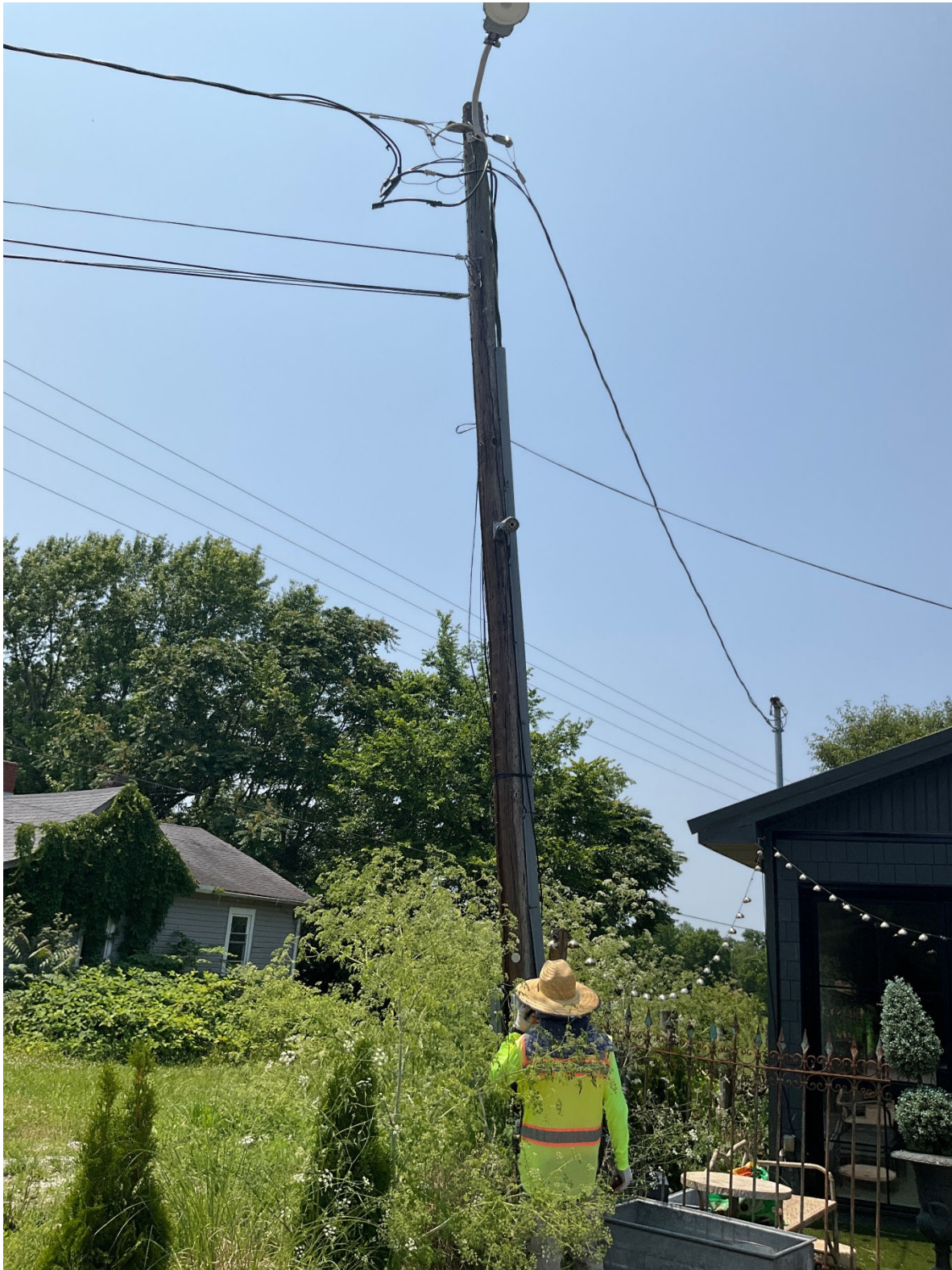
Figure 5.2 – Communications attachments are above the top of the electric service riser in the power space.
